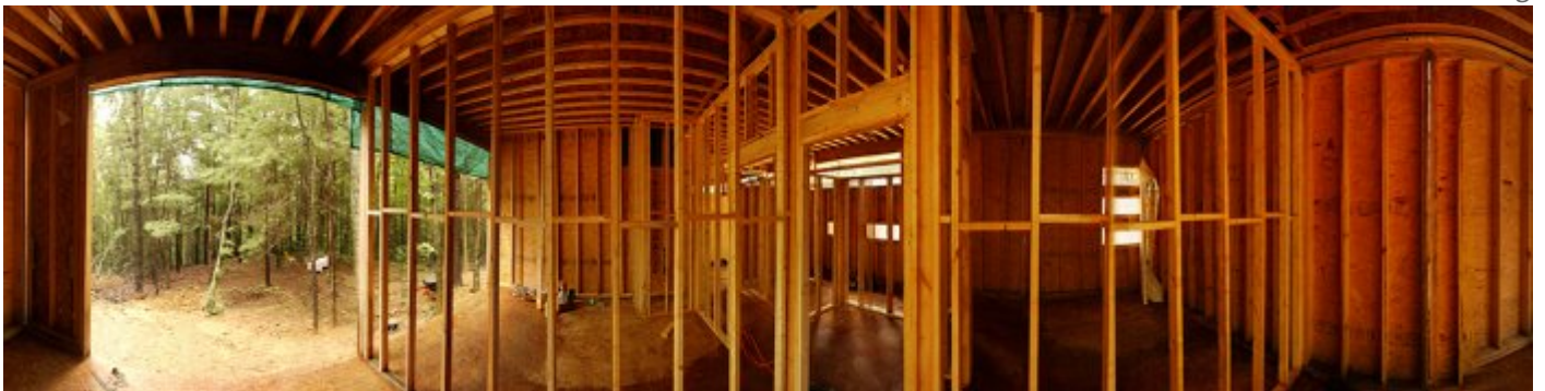
Below: interior of LV home after framing
